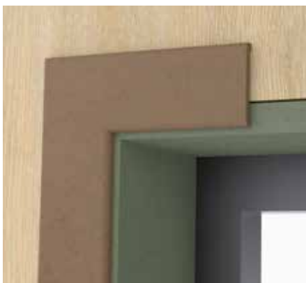
Window finish with MDF and window frame
